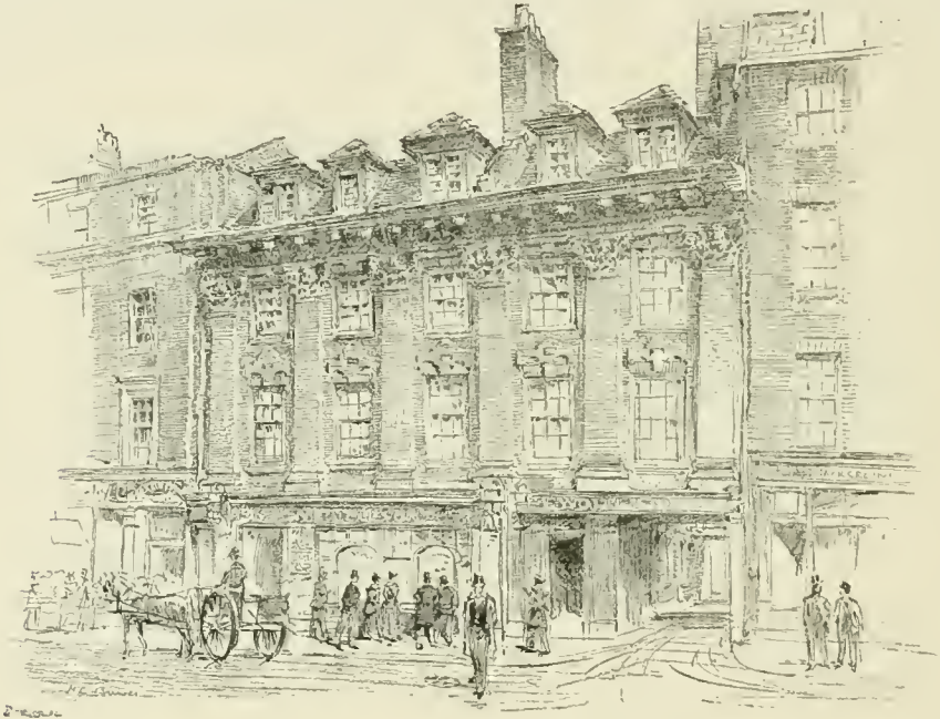
OLD HOUSES IN GREAT QUEEN STREET.
